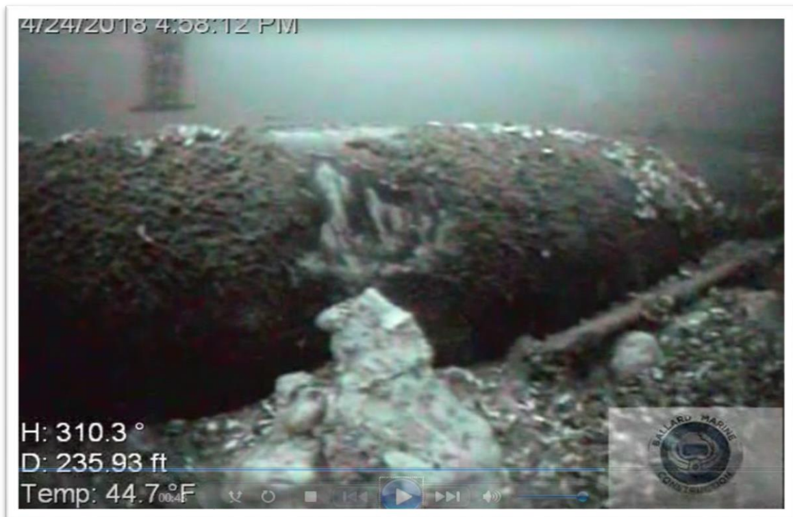
Figure 4-14 Dent and impact marks west pipeline. ROV imagery provided by Enbridge Inc.
