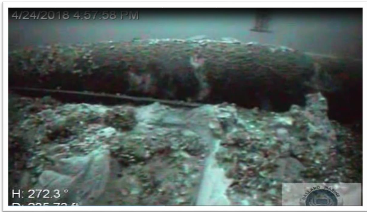
Figure 4-15 Gouges in Enbridge's west pipeline. ROV imagery provided by Enbridge Inc.
